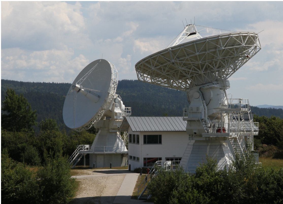
Figure 6.4: The Wettzell Twin Telescope with its two 13.2 m antennas (Wn in the front) and the control building.
