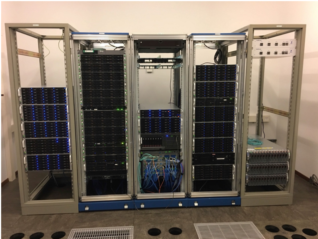
Figure 7.3: New correlator and network hardware during installation at JIVE.
