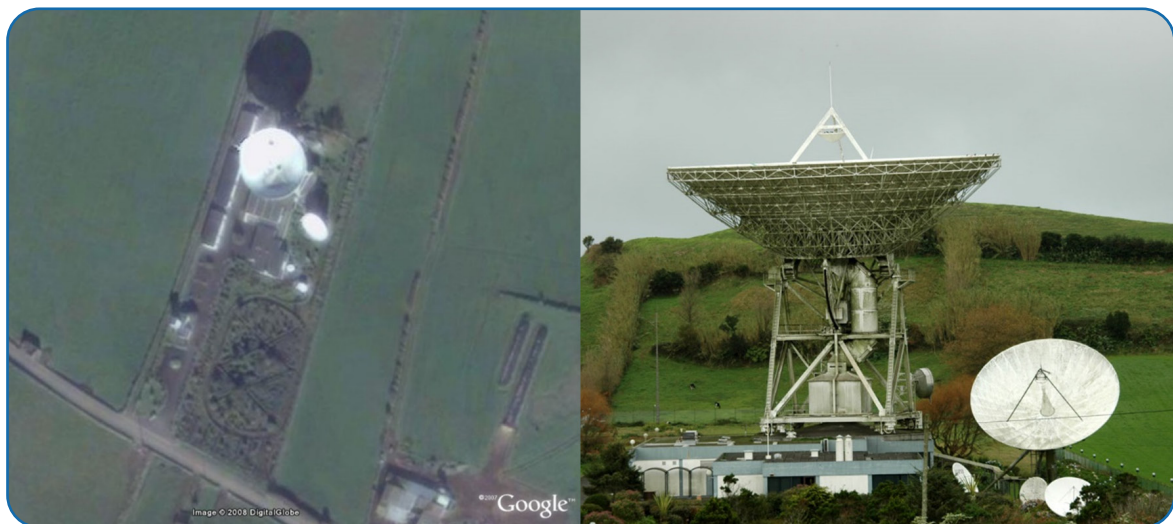
Figure 1: SATCOM Earth Station in São Miguel (Azores) - Intelsat Standard A 32-metre parabolic antenna, Altice Portugal. We can see the typical large waveguide system below the dish.
