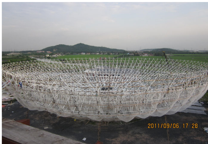
Figure 1: Shanghai 65-Meter Radio Telescope. (top): The mount of the telescope has been completed. (bottom): The assembly of the primary reflector structure has been finished on the ground and will be installed on the alidade of the telescope late this year or early next year.
