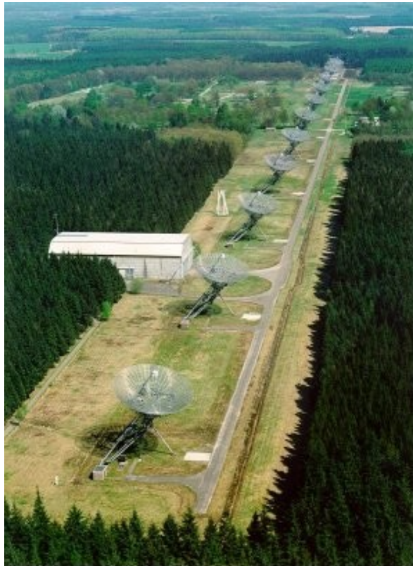
The Westerbork Synthesis Radio Telescope (WSRT) consists of 14 dish-shaped antennas
