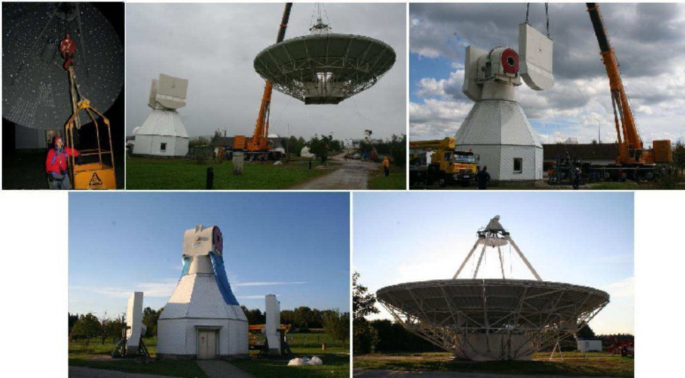
Repair of the bearings of the 20-m radio telescope.
