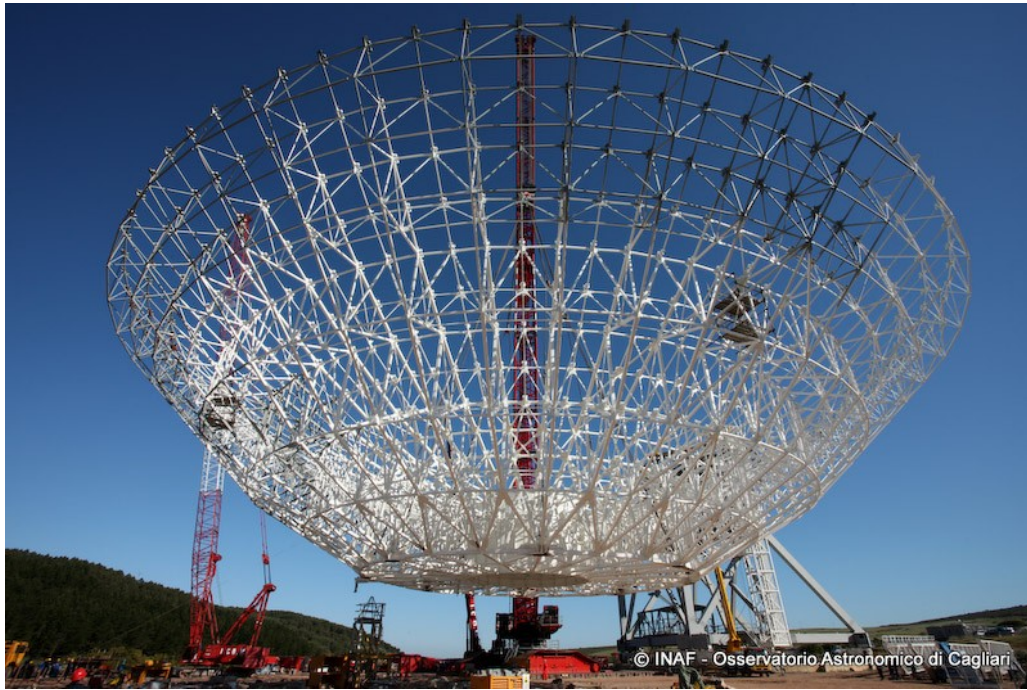
Fig. 1 Installation of the primary mirror back-up structure
