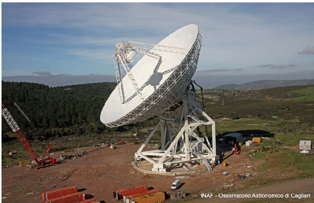
Fig. 2 SRT structure completed and moving
