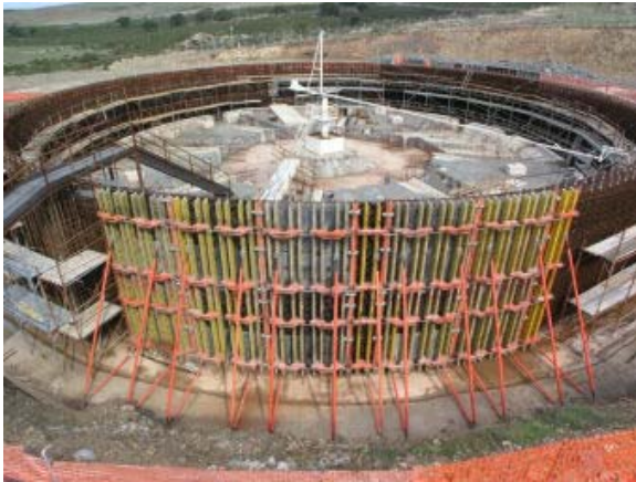
Fig. 3 - The Sardinia Radio Telescope foundation in October 2004.
